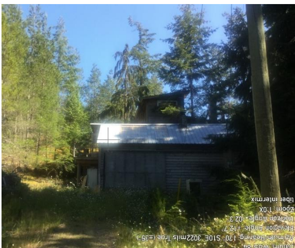
Figure 6. Intermix structures with wood siding and combustible material stored within ignition zone, typical throughout the AOI.
