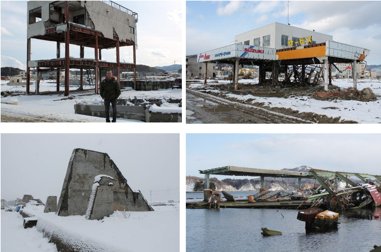
Figure 24. Damaged infrastructure in the City of Miyako, Japan following the 2011 Tohoku tsunami (Photos: Philippe St-Germain/NHC, 2012). Top photos show damage to inland buildings, bottom left photo shows remains of tsunami protection wall, and bottom right show damage to port installations.
