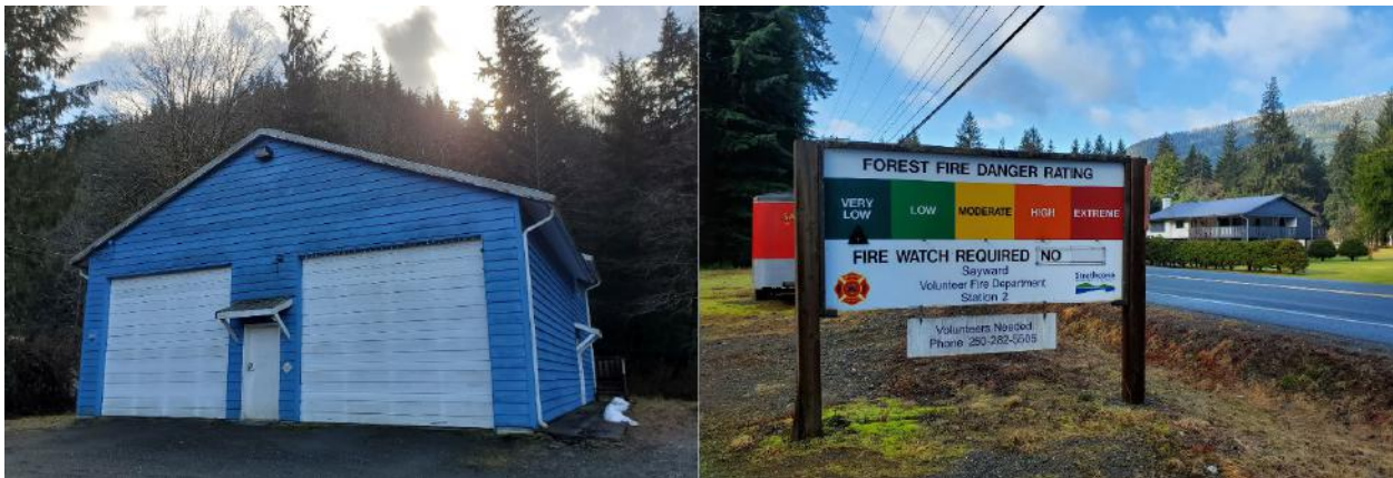
Photo 4. Sayward Volunteer Fire Department Firehall No. 2.
