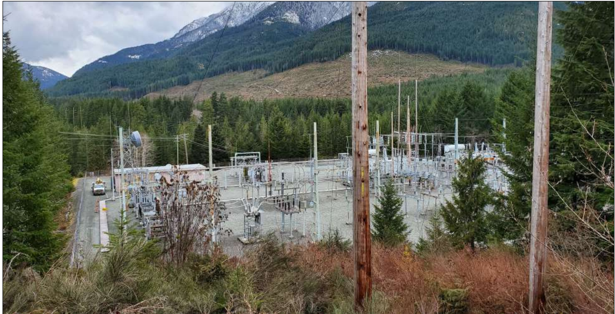
Photo 4. View of BC Hydro Substation from Gold River Road.
