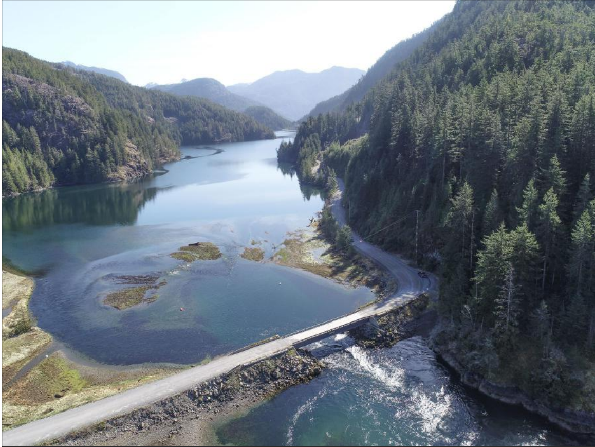
Photo 7. Fair Harbour FSR and the causeway bridge crossing Little Espinosa Inlet.
