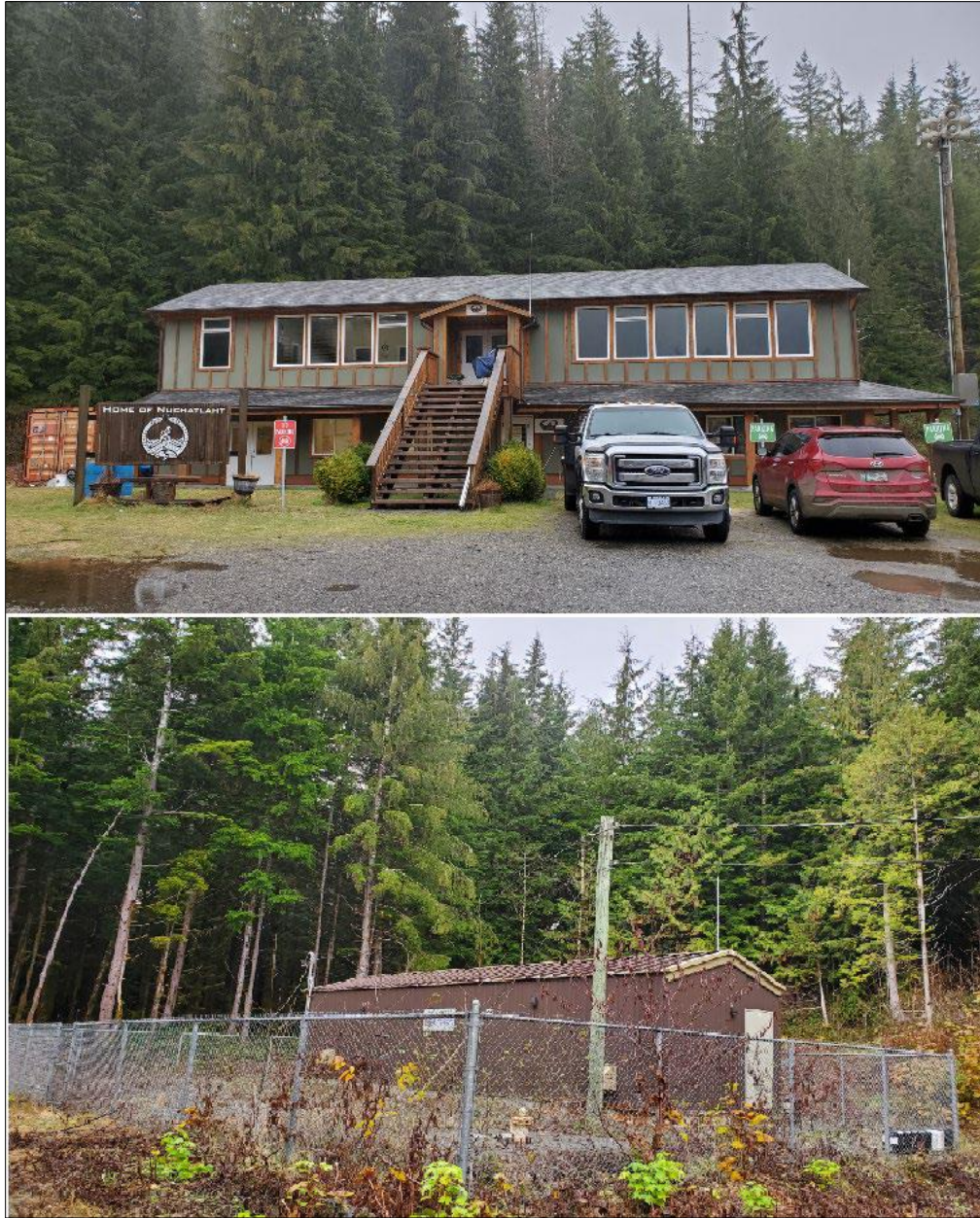
Photo 2. Nuchatlaht First Nation Office above, and water treatment plant below.
