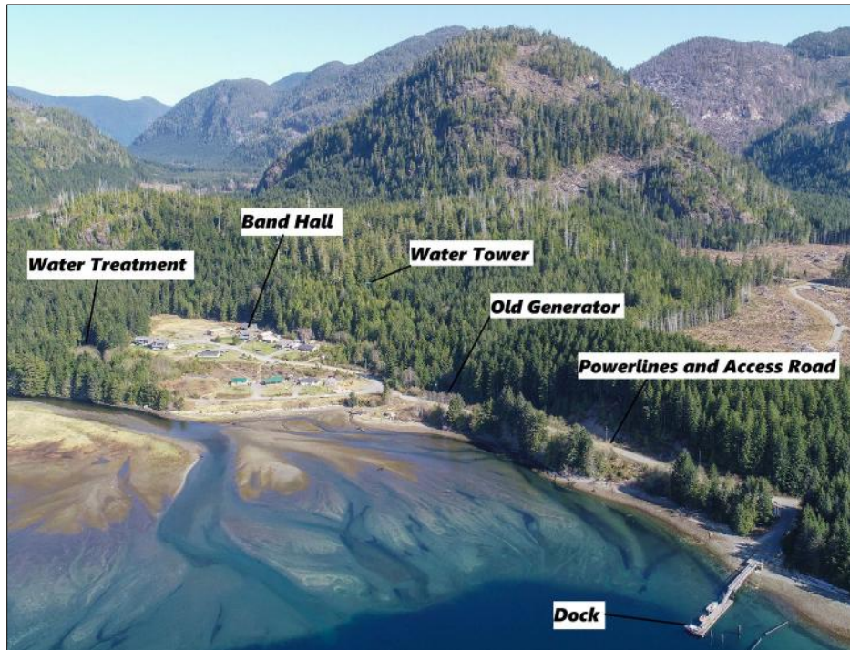
Photo 1. Aerial image of critical infrastructure in Oclucje.
