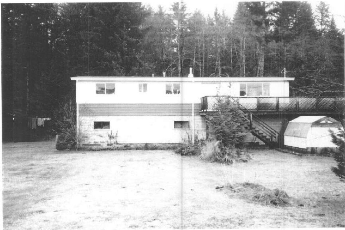
PHOTO 6: VIEW OF KNUTSON HOME ON GLENROY ROAD NOW FLOODPROOFED (REFER TO HWM 90-25/26)
