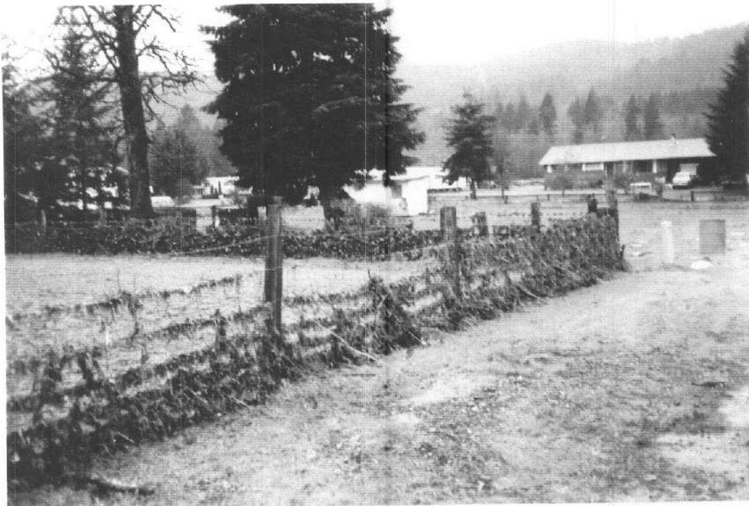
PHOTO 4: LOOKING TOWARD HWM 90-29 ARMISHAW ROAD IN THE VICINITY OF XS 17/18 NOTE DEBRIS ON FENCE
