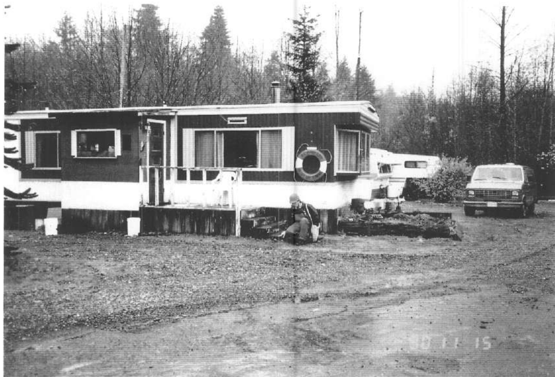
PHOTO 7: HWM 15/16 - ADJACENT TO FCL 7.0m HWM FROM OVERLAND FLOW
