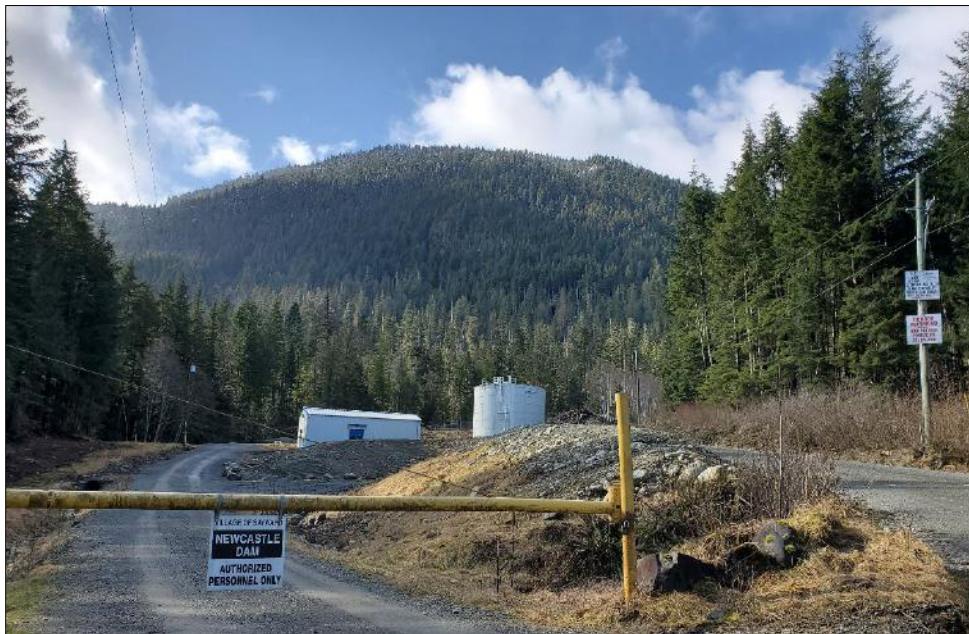
Photo 3. Water treatment facility and storage reservoir.
