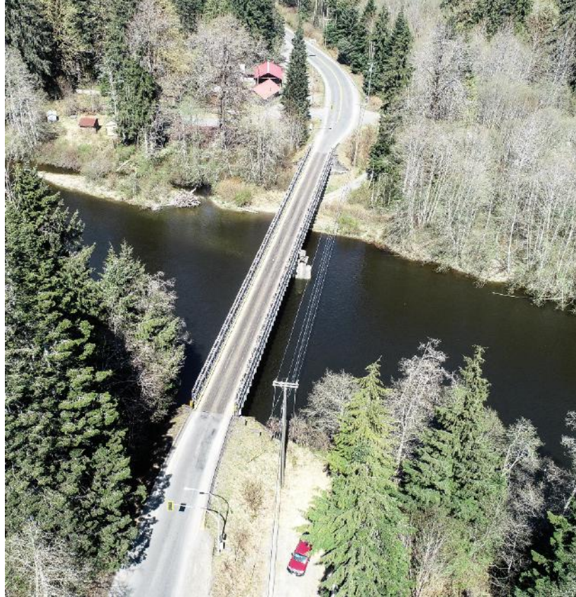
Photo 10. Potential bottleneck for emergency evacuation – single lane bridge on the Salmon River.
