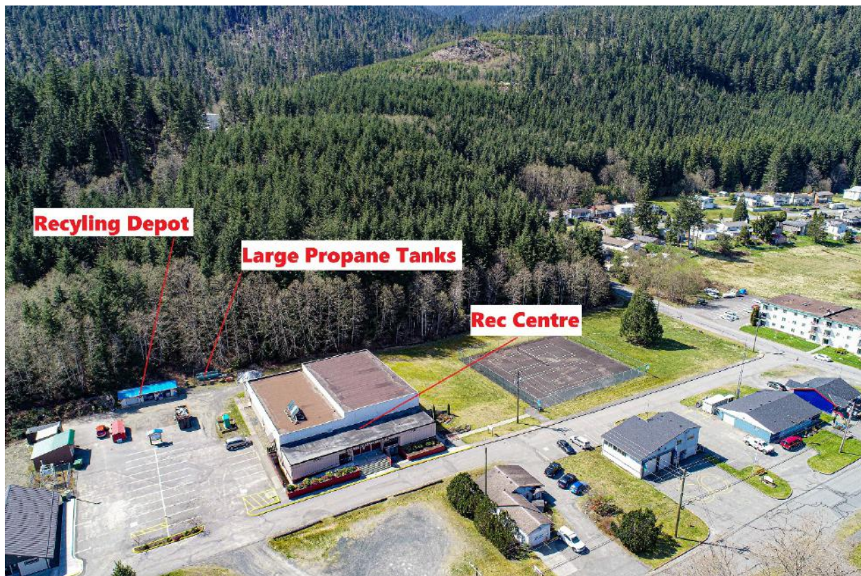
Photo 4. Recycling Depot and Propane Tanks behind the Rec Centre.
