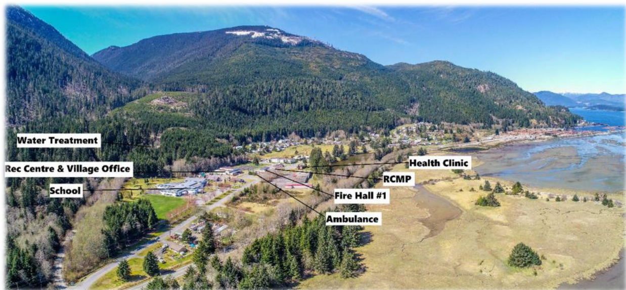
Photo 2. An aerial overview of Sayward's critical infrastructure.
