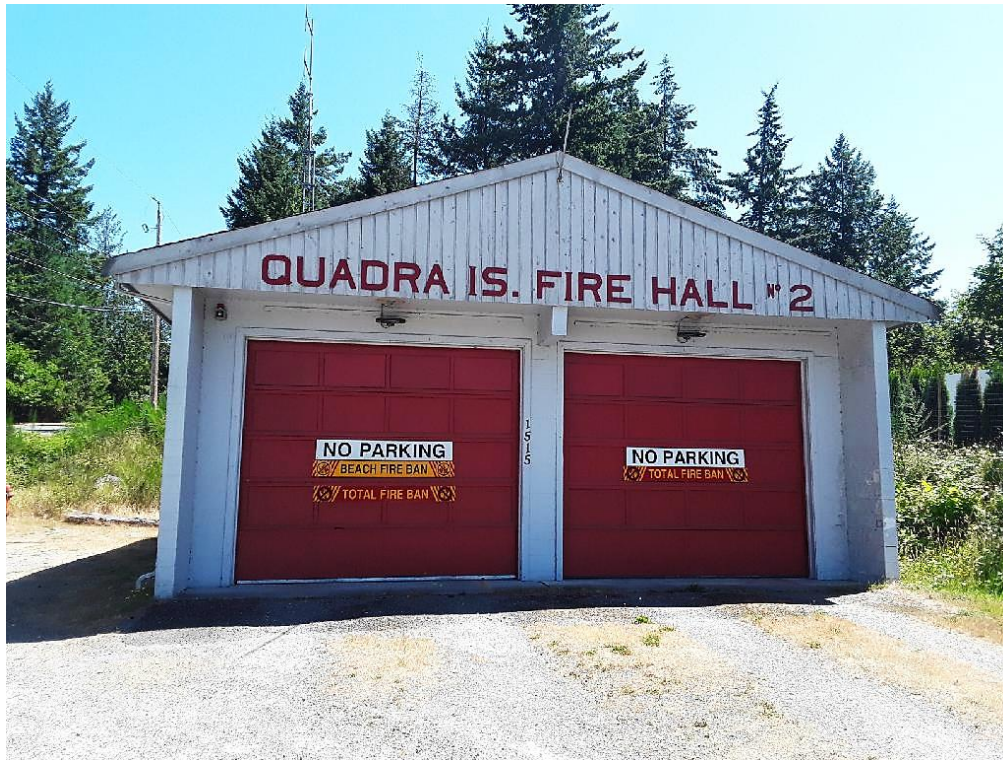
Figure 4: Quadra Island Fire Hall #2
