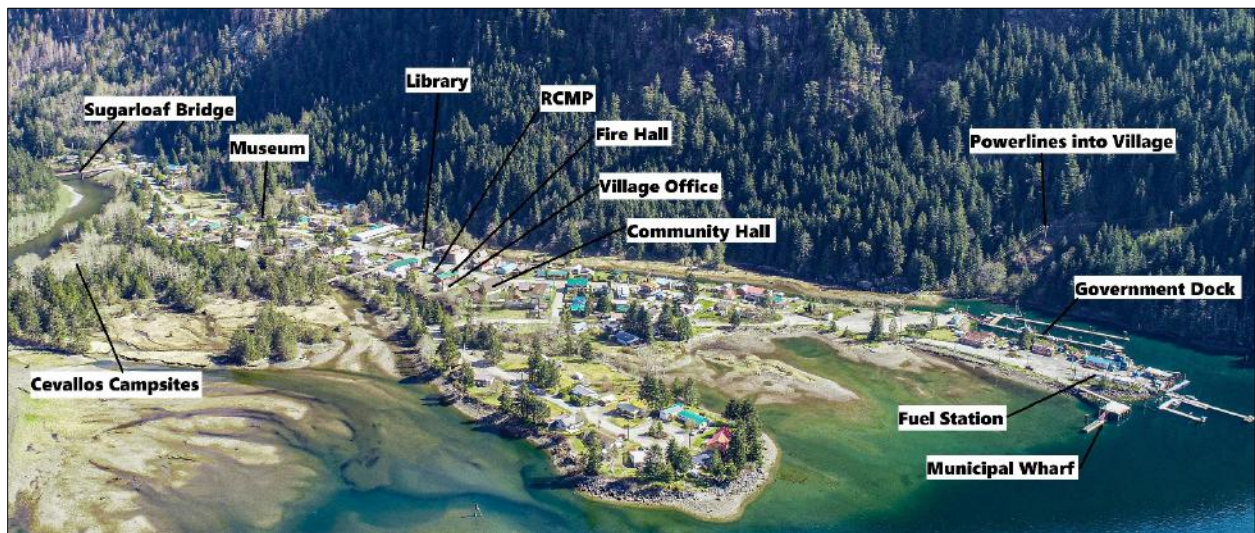
Photo 4. Critical Infrastructure east of Sugarloaf Bridge.
