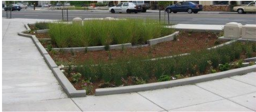
Bioretention area utilizes water from the adjacent road surface. (Source: Abby Hall, US EPA).
