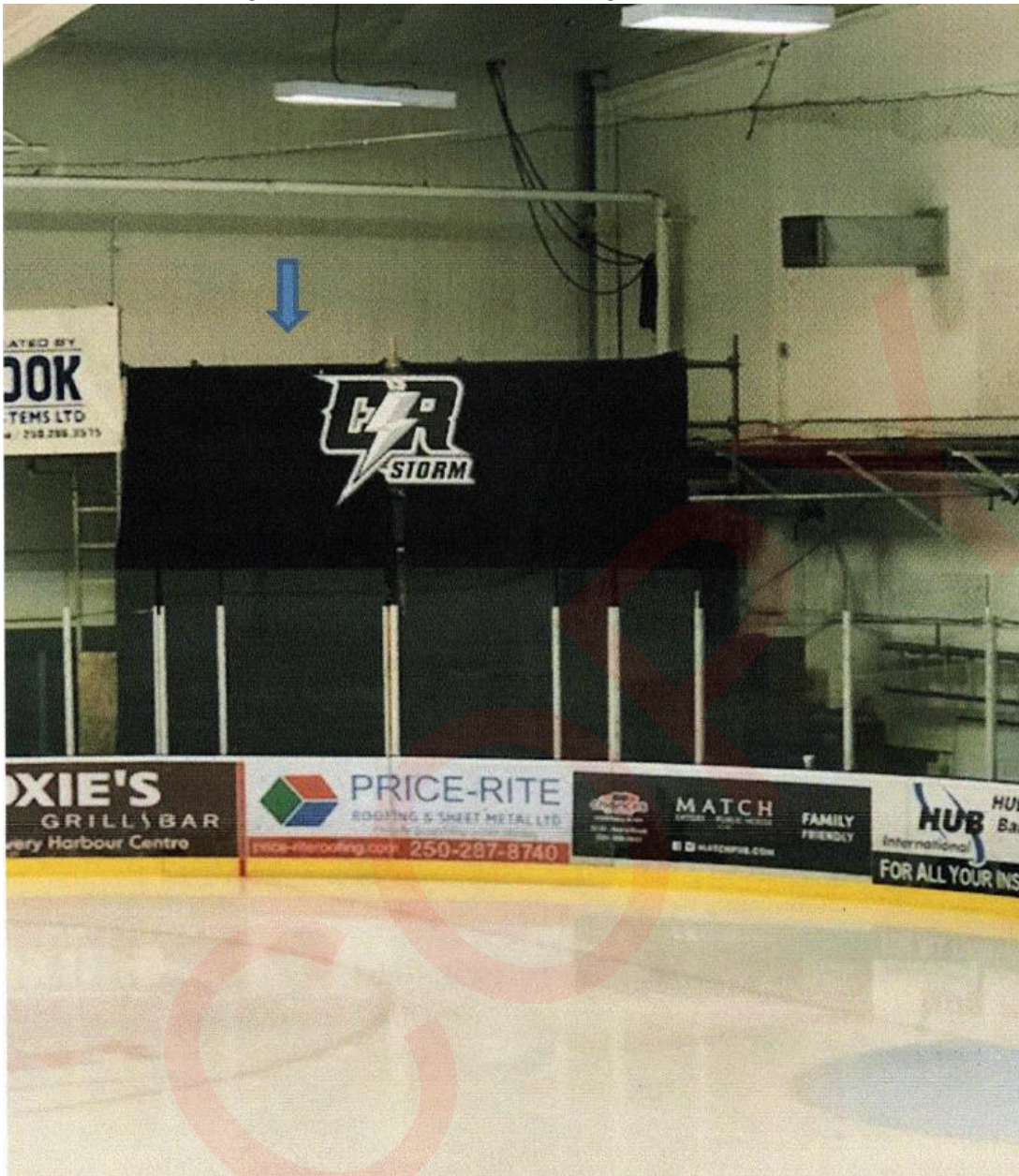
EXHIBIT 2 – Scaffolding located outside of Storm dressing room.
