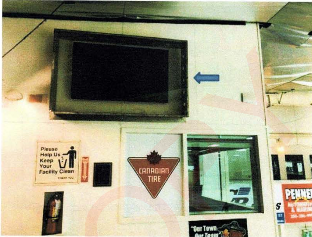
EXHIBIT 1 – Campbell River Storm VIP north signage and television monitor with metal protective casing.
