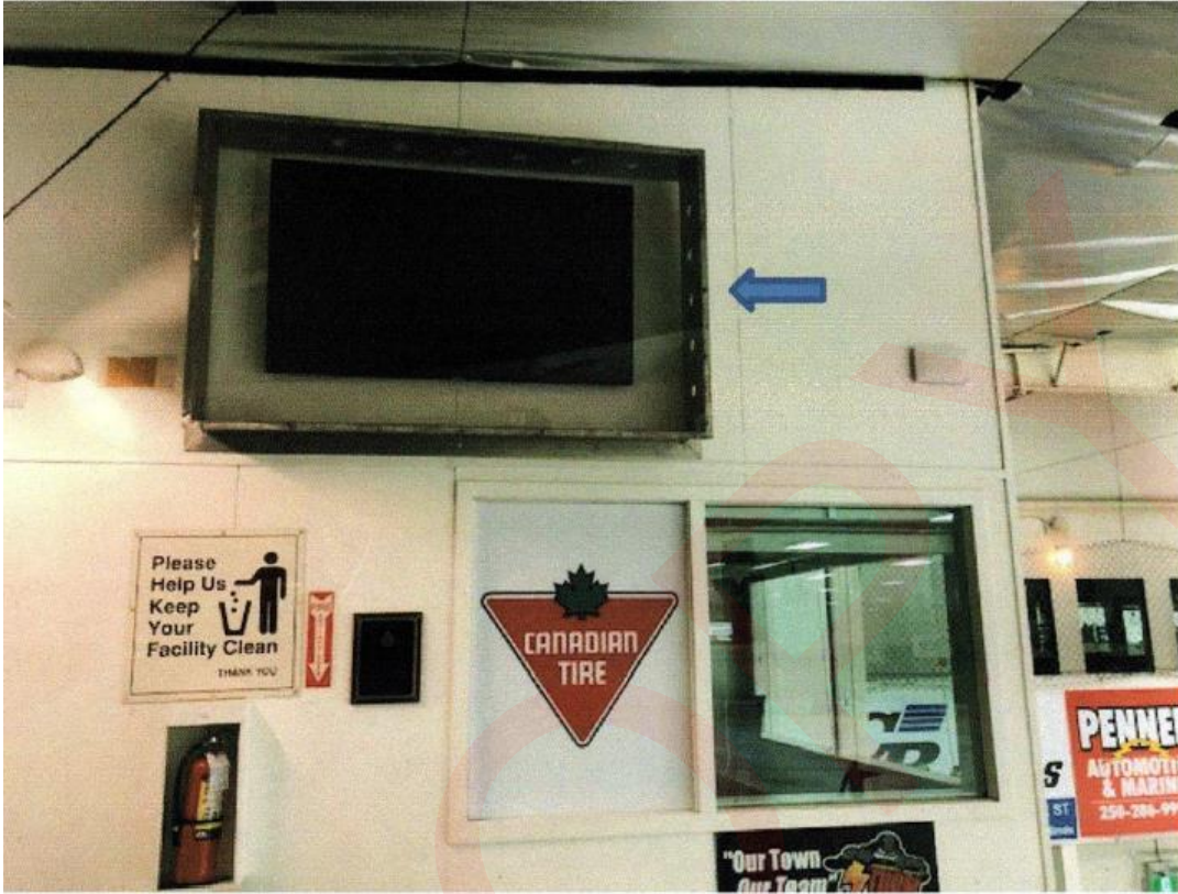
EXHIBIT 1 – Campbell River Storm VIP north signage and television monitor with metal protective casing.
