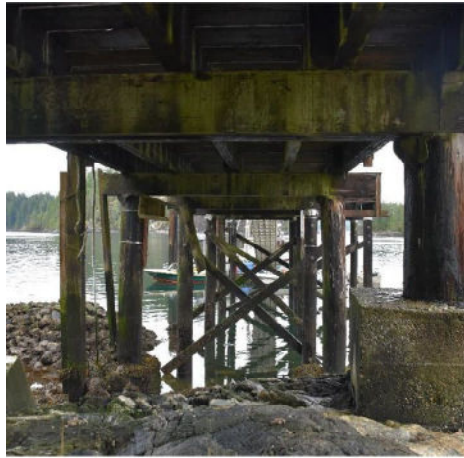
Figure 2 – Typical configuration of wharf piles and cross-bracing.
