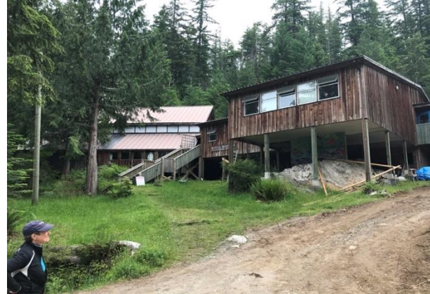
Figure 3. Surge Narrows School
