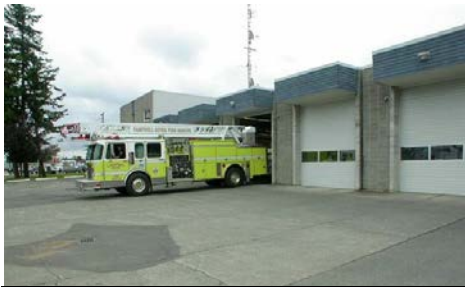
Campbell River Firehall #1 (Photo courtesy of Campbell River Mirror)
