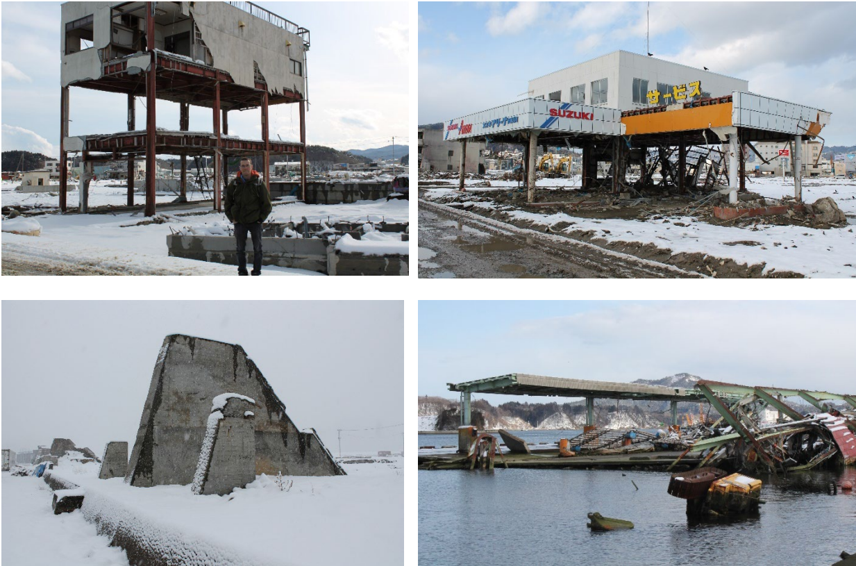
Figure 24. Damaged infrastructure in the City of Miyako, Japan following the 2011 Tohoku tsunami (Photos: Philippe St-Germain/NHC, 2012). Top photos show damage to inland buildings, bottom left photo shows remains of tsunami protection wall, and bottom right show damage to port installations.
