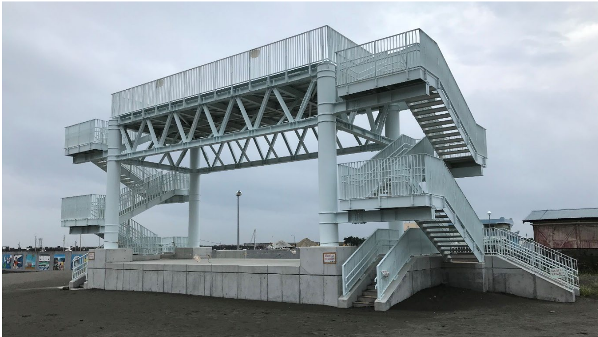
Figure 29. Tsunami vertical evacuation tower near Kamakura, Japan (Photo: Philippe St-Germain/NHC, 2018)
