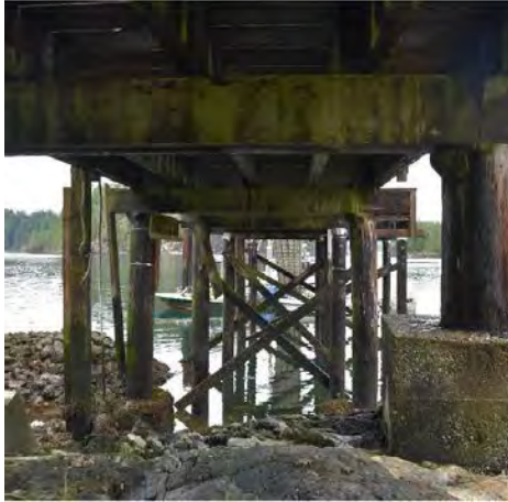
Figure 2 – Typical configuration of wharf piles and cross-bracing.
