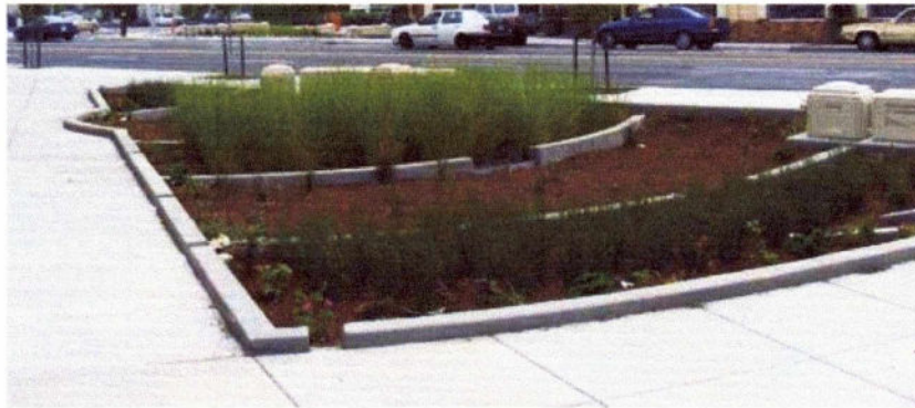
Bioretention area utilizes water from the adjacent road surface. (Source: Abby Hall, US EPA).
