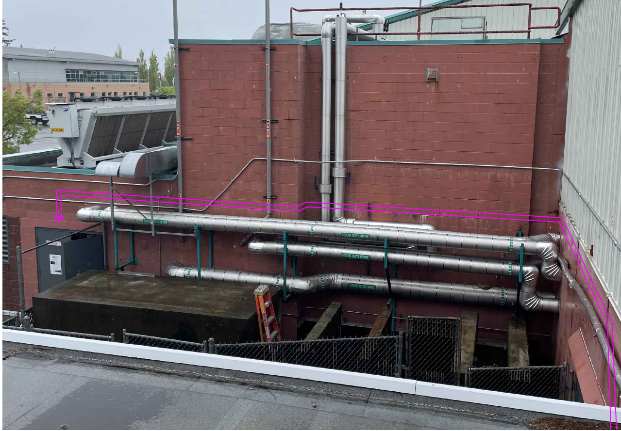
3 M7 EXTERIOR PIPE RUN 1. ROUTE NEW HC1 PIPING ALONG EXTERIOR WALL. 2. COORDINATE WITH EXISTING PIPING AND EQUIPMENT.
