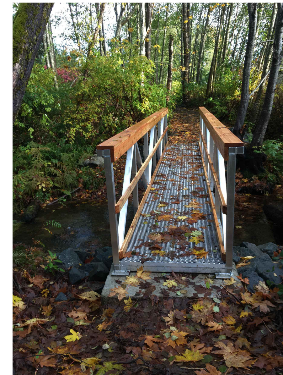
PHOTO: TIMBER DRESSING
